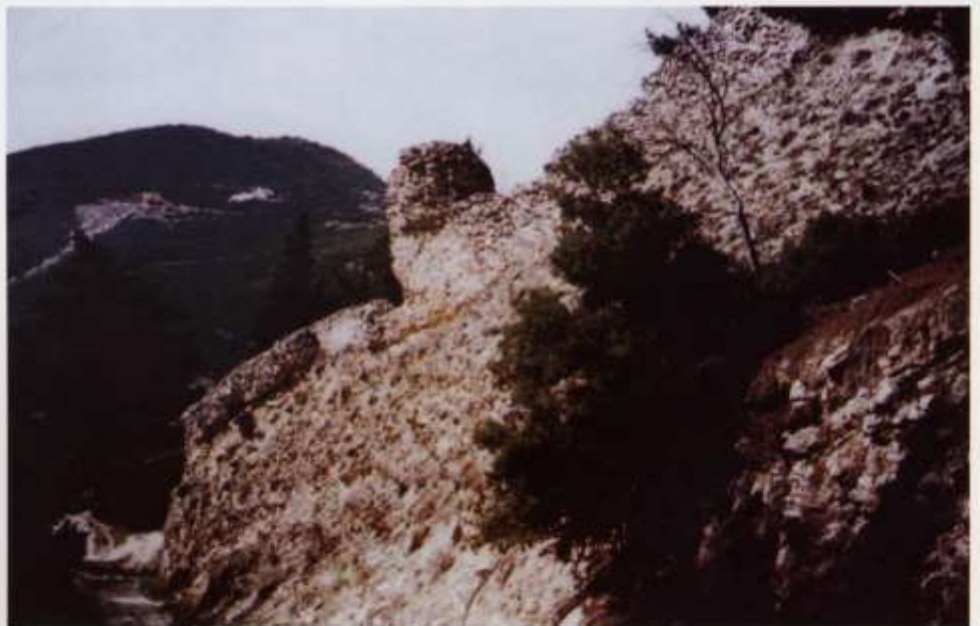
figure 25: Southeast part-Inner enclosure. Most of the external part (first phase) has collapsed.
