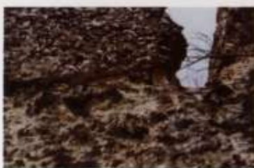
figure 26: Southeast part-Inner enclosure. External façade. Detail of the demolished foundation.
