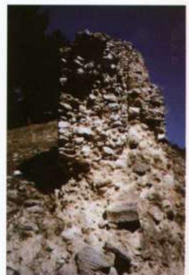
figure 10: Inner enclosure. Southeast part. The two different phases. The inner part was probably constructed later to increase the thickness of the wall.
