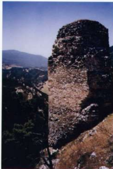
figure 19, 20: Acropolis. Massive tower. Ground problems and demolished masonry at the lower and upper parts.
