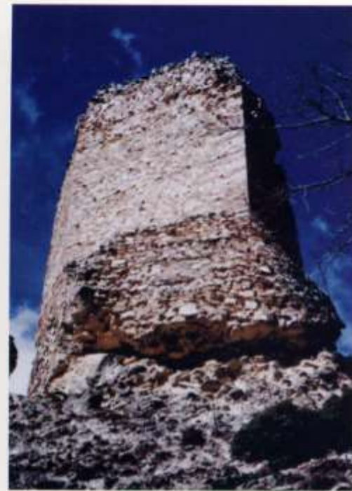
figure 4: The massive tower of Acropolis. The lower part belongs to the first phase and the upper to the second.
