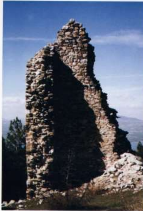
figure 17: Acropolis Northwest tower. After the earthquake in 1995.
