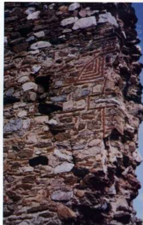
figure 5: Northwest rectangular tower. Detail of brick decoration.
