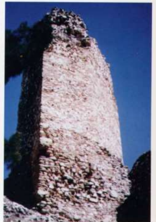
figure 19, 20: Acropolis. Massive tower. Ground problems and demolished masonry at the lower and upper parts.
