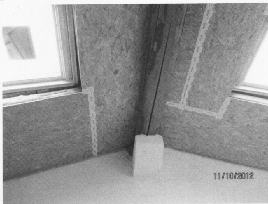
Figure 1. Insulation at the internal façade of the external walls.
