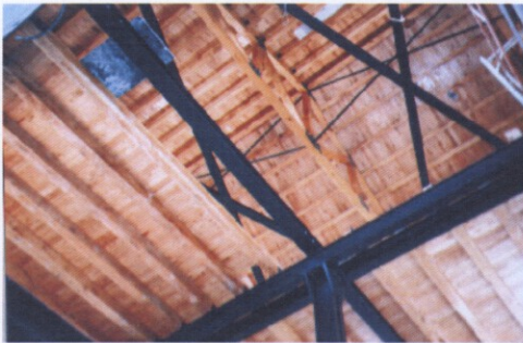
Figure 3 Reconstruction of metal carrying system, timber floors and roof
