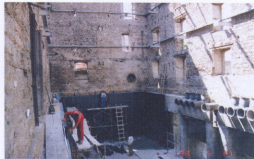
Figure 4 The construction of a basement in the mill
