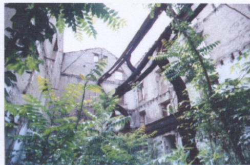
Figure 2. The internal space before the restoration works
