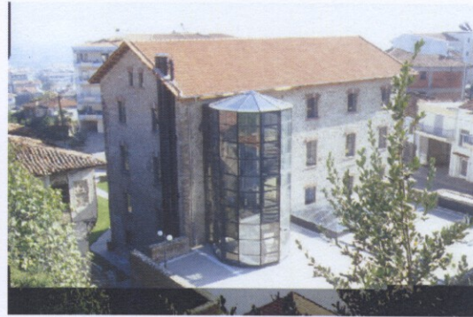
Figure 7 The external staircases and the roof of the atrium
